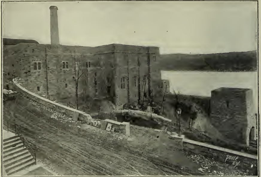
FIG. 2. VIEW OF POWER PLANT FROM THE ROAD
